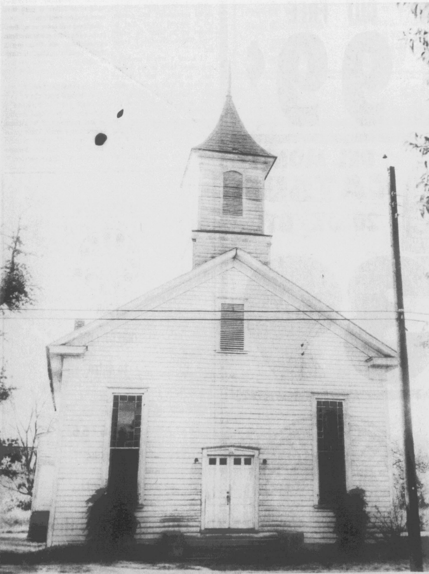
"THE FINEST CHURCH IN THE COUNTY." . . when it was built as a result of a revival in 1877, featured stained glass windows, a bell tower, lighting rods, and weather vanes, and a chandelier with 12 kerosene lamps. The building first housed the Bethel Methodist Church, from which the town is named. It is now Medley Chapel C.M.E. Church.
