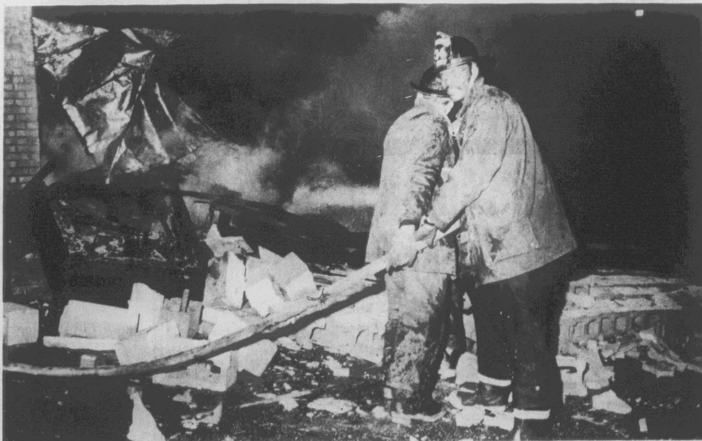
MAN DIES IN BLAZE . . . Greenville Firemen bring a fire under control last night at the Mark IV Club on Albemarle Ave., which killed a still, unidentified man. Firemen reported the building
