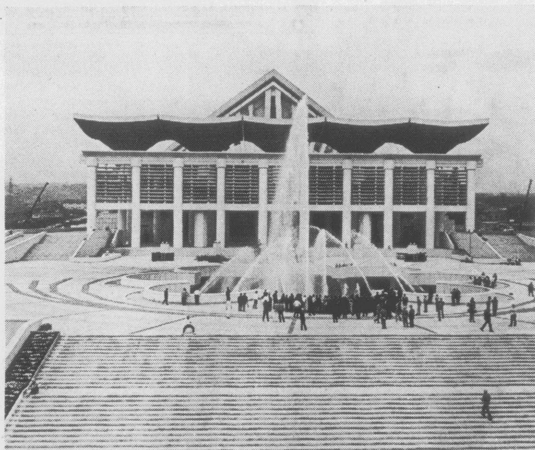
Front of Sho-Hondo. In foreground is the Garden of the Law with sunken fountains.
