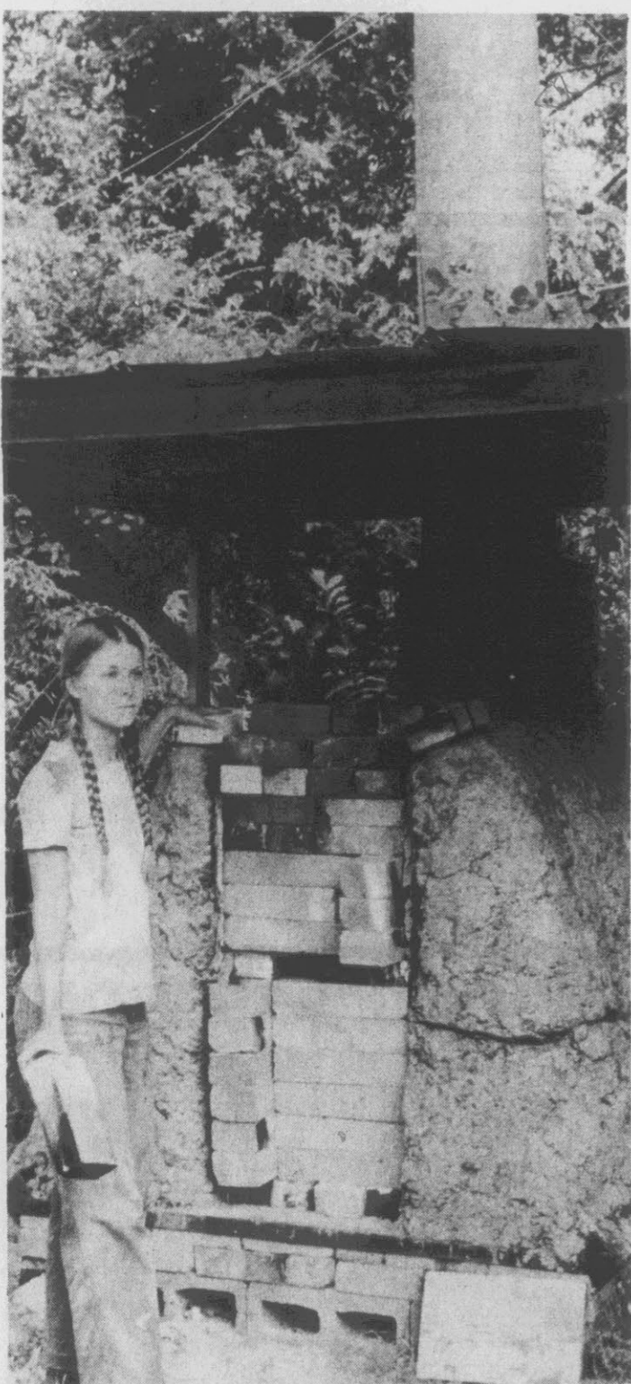
HOME-MADE KILN. . . was constructed by Miss Cynthia Ryals of Greenville from scrap brick and then covered on the outside by adobe made from clay and sawdust.
