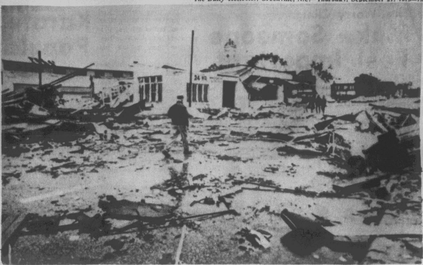
MAIN STREET IN RUBBLE — Residents of Clay Center, Kansas, found a large portion of their downtown area in rubble town's main street about 8:05 p.m. Tuesday. The twister was one of several touching down in north-central Kansas Tuesday night. (AP Wirephoto)
