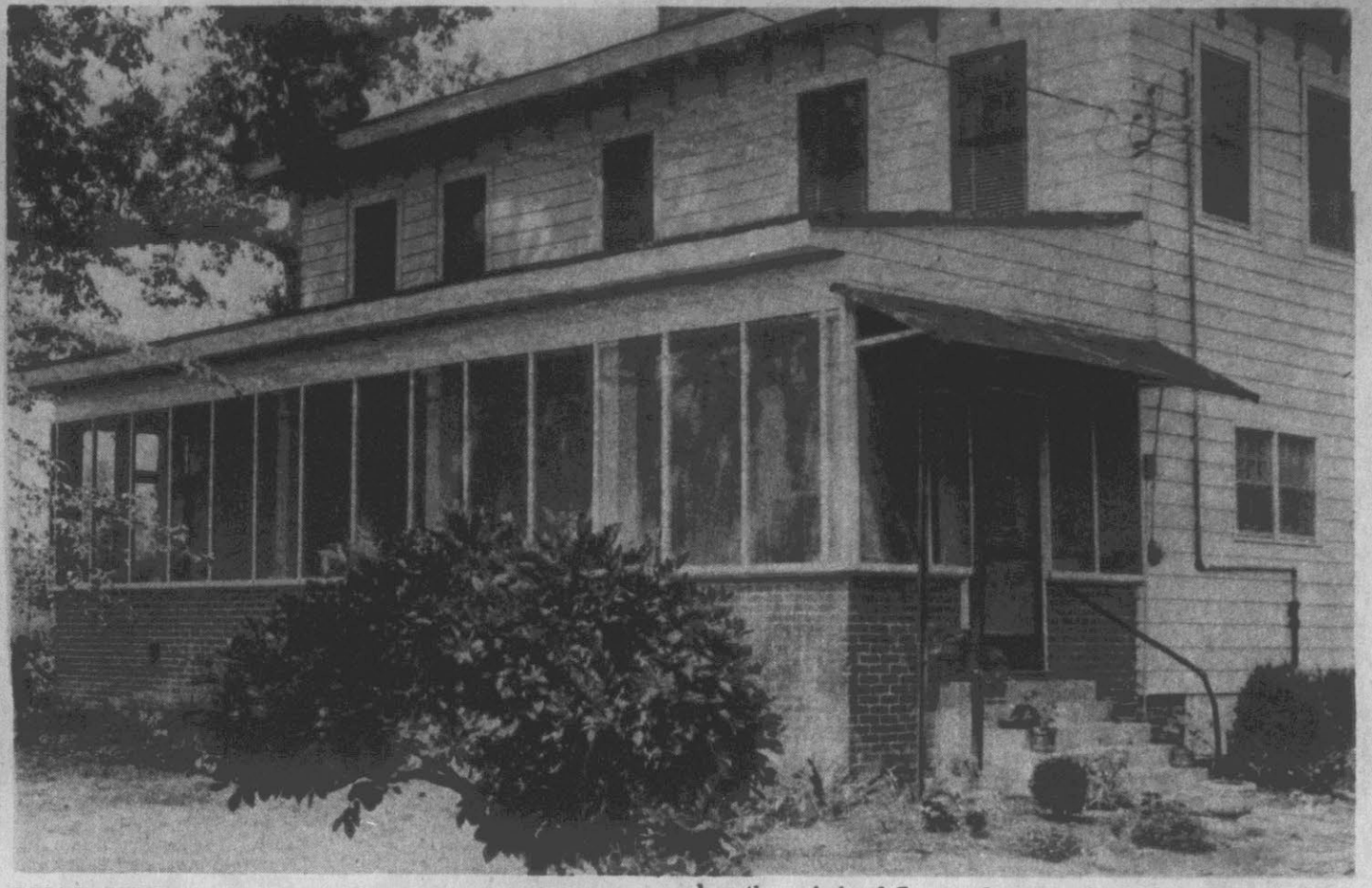
REAR VIEW . . . of the Brooks home shows the spacious back porch that was added in 1919. The home
