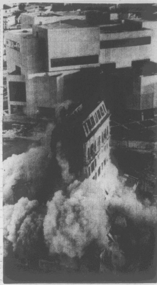
GONE IN A CLOUD OF DUST —A nine story structure was demolished in less than a minute Sunday morning on Second Avenue in Miami. The building, built in the early 1920s was demolished by explosives in the early morning while few people were in the downtown area. In the background is the new downtown campus of Miami Dade Junior College. (AP Wirephoto)
