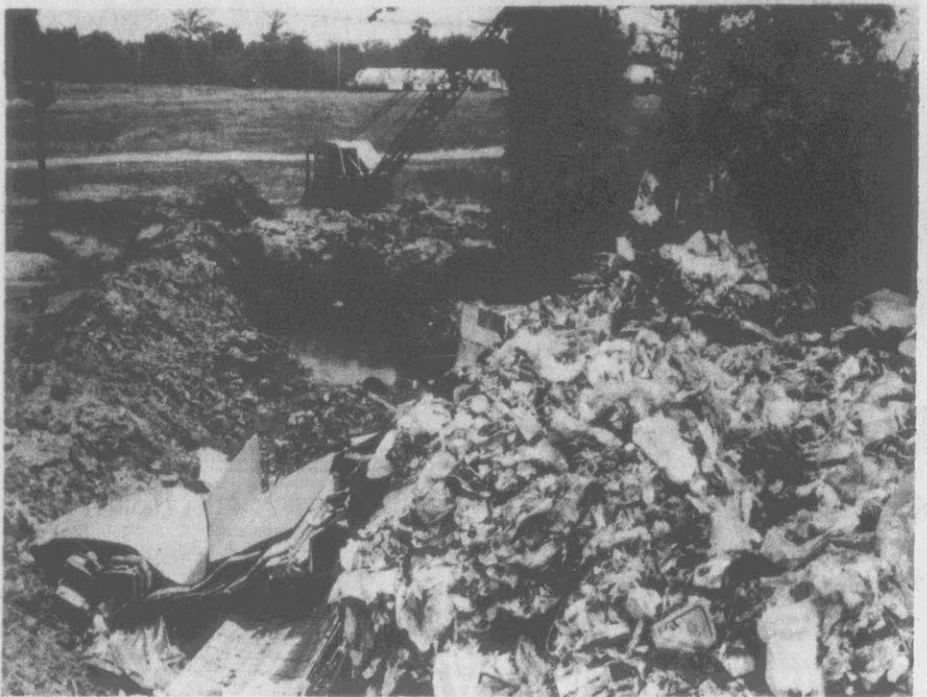
TEMPORARY LAND FILL AREA . . . near East Second Street is shown in these two photographs. The top photo shows the first area already
