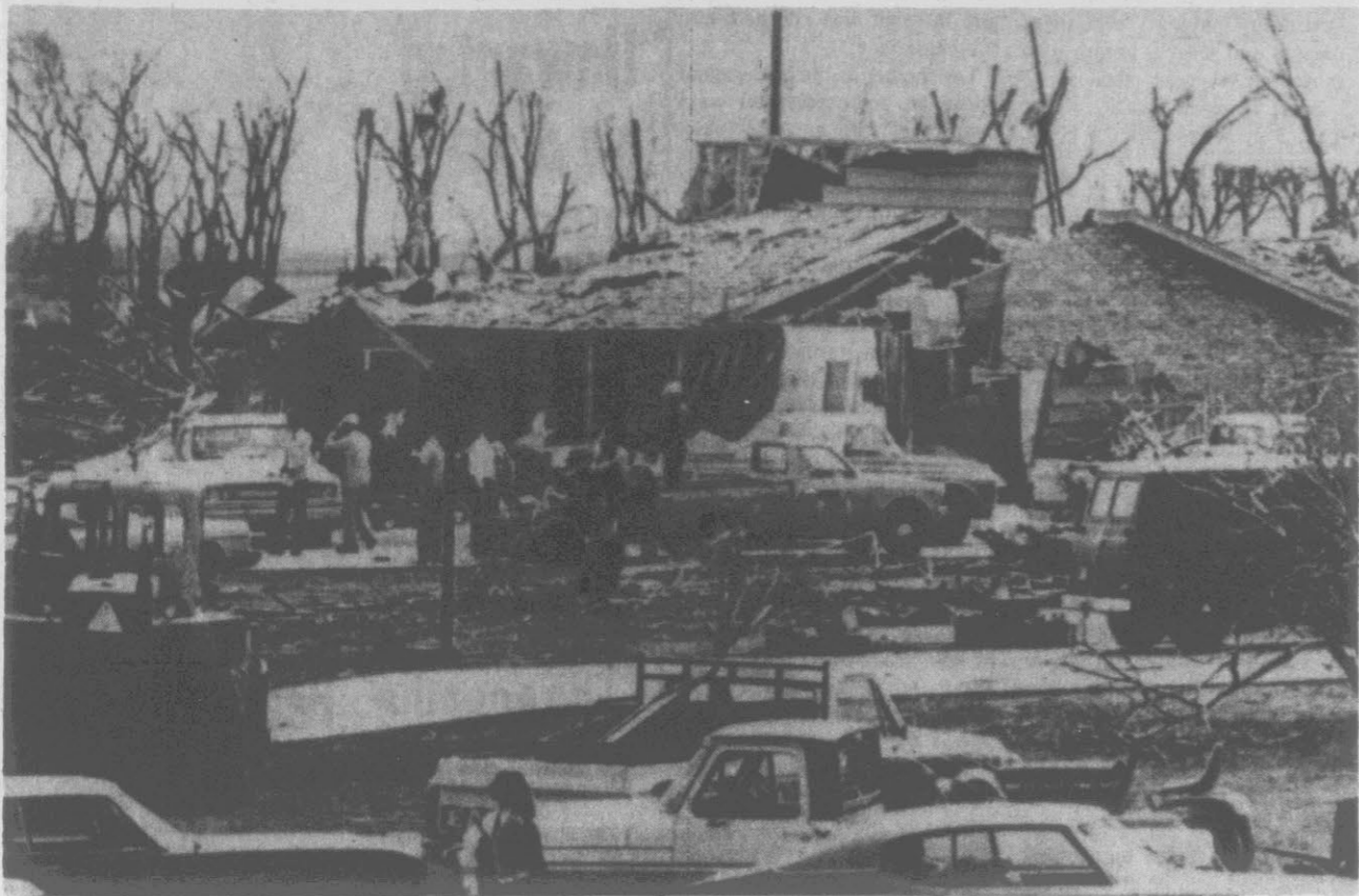
TORNADO CLEANUP —Residents and friends came from all around to help those whose homes were destroyed in a killer tornado which struck Plainview Texas early Sunday morning. The home above was located in the fashionable Westridge section of Plainview. (AP Wirephoto)
