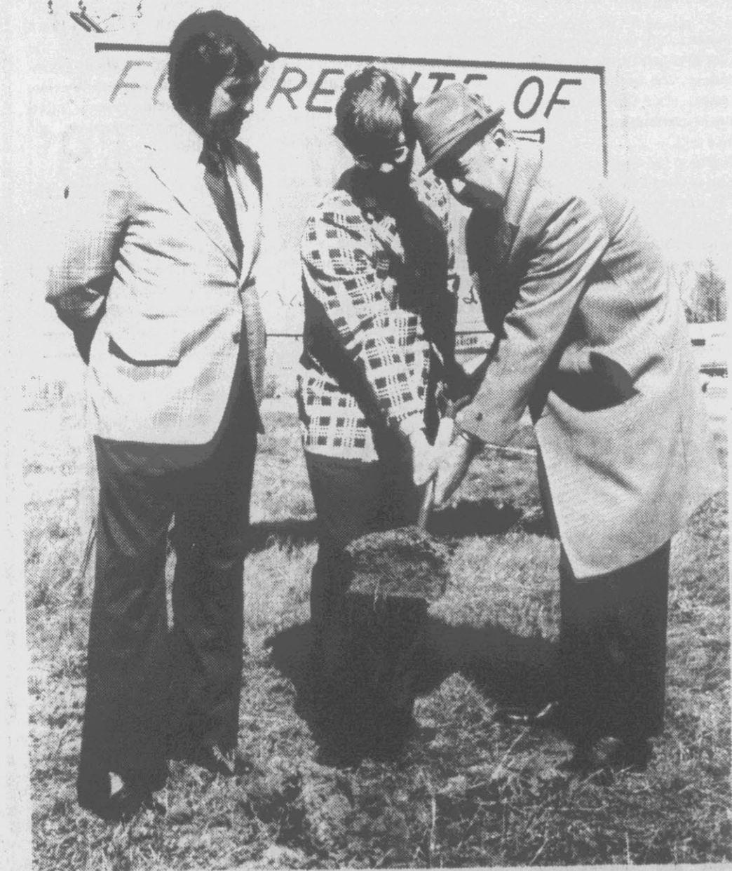
BREAKING GROUND. . . Ground was broken for the new Ramada Inn to be constructed on the 264 By-pass near the Pitt Plaza shopping area yesterday. Breaking ground is Marvin Buck, part owner (center) and Greenville Mayor Eugene West (right). Ed Dupree, project
