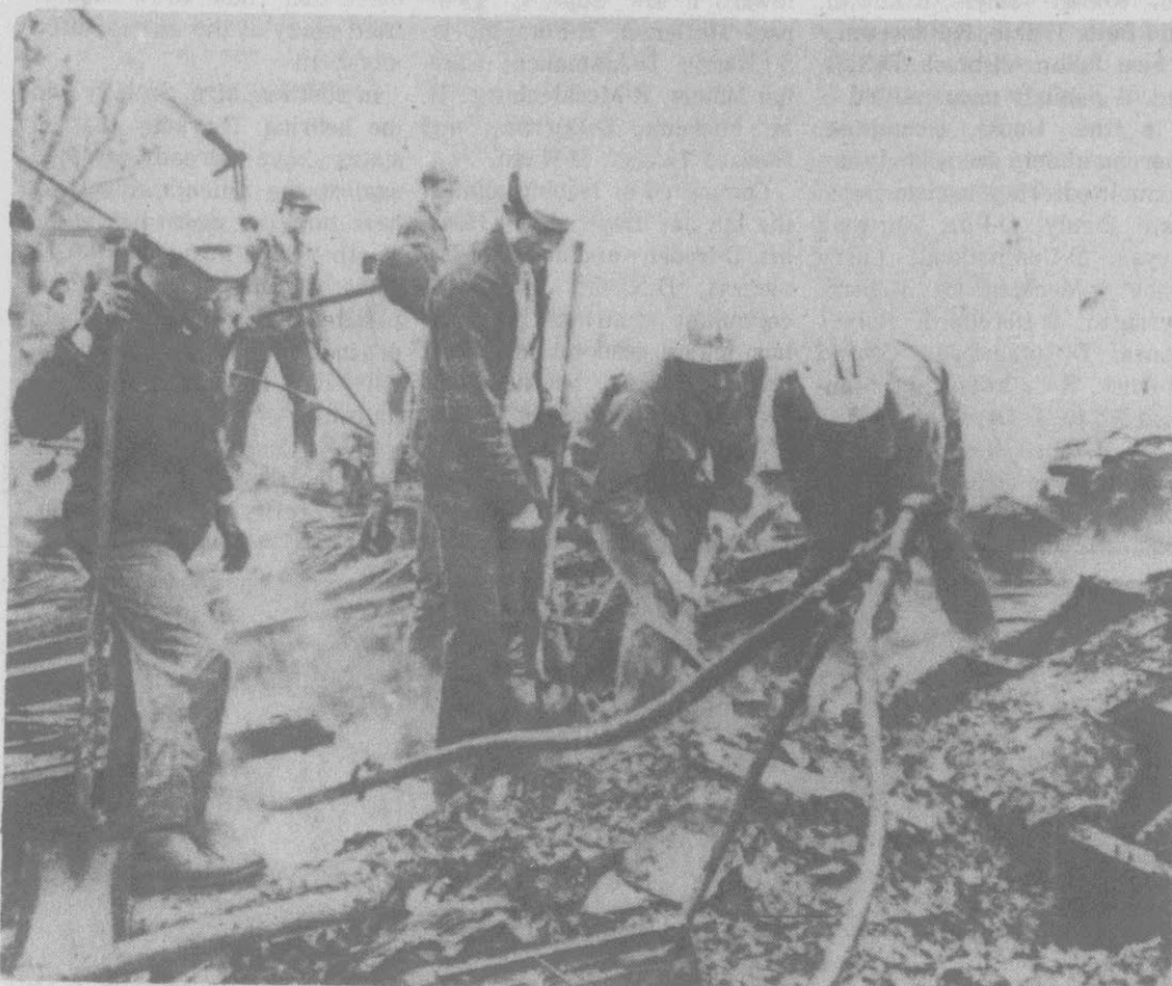
THE SEARCH GOES ON — A Navy jet fighter plane crashed into an apartment building Wednesday night in Alameda, Calif., and rescue workers continue to sift the debris, searching for possible victims. (AP Wirephoto)
