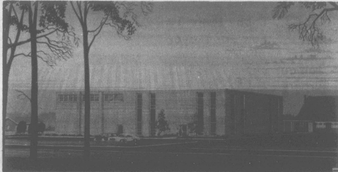
Educational Building Now Under Construction J. H. Hudson, General Contractor
