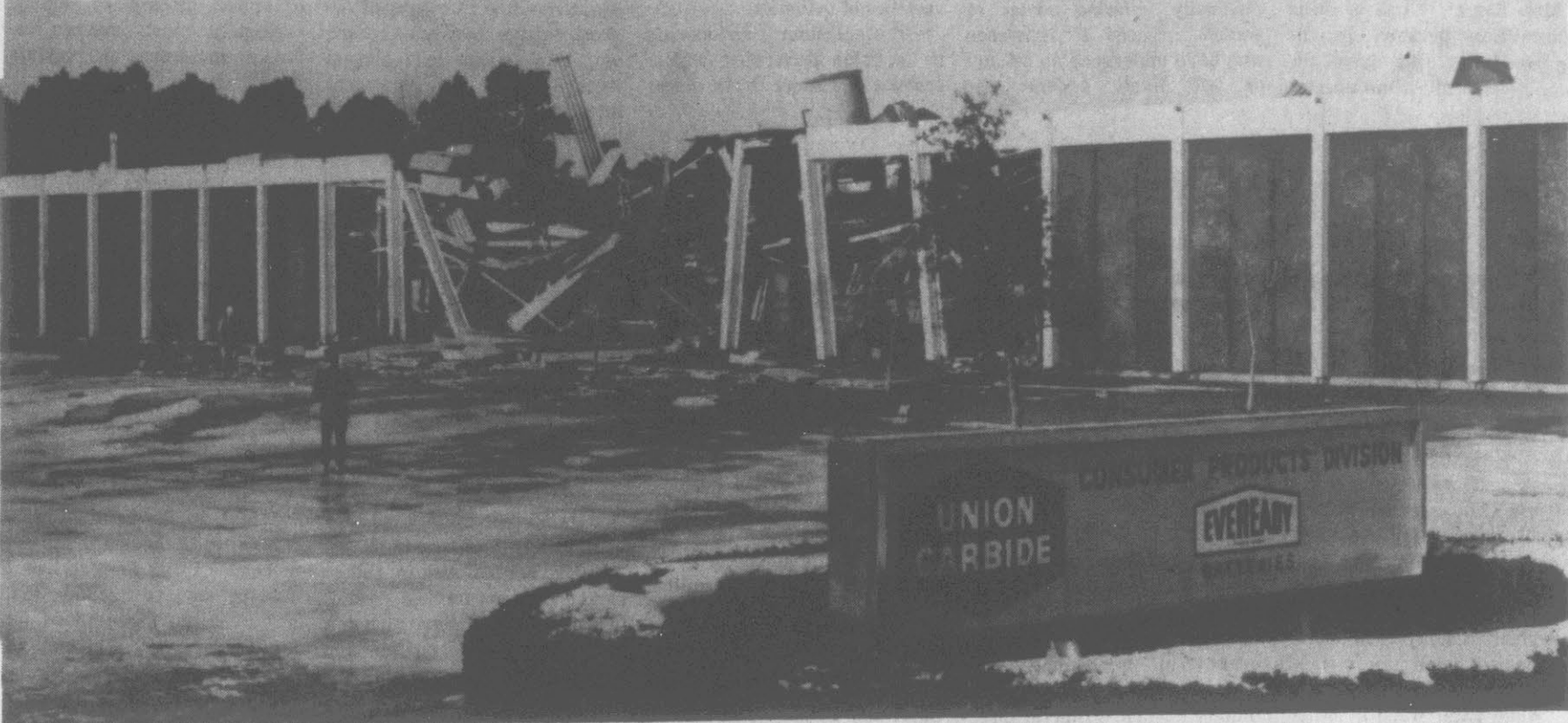
PLANT DAMAGED... The Union Carbide plant at the intersection of Evans Street and U.S. 264 was heavily damaged early Sunday morning when a gas fired steam boiler exploded, sending one
