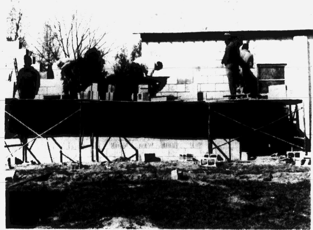
MASONRY INSTRUCTION . . . Masonry students at Pitt Technical Institute gain valuable and practical experience by performing needed public services such as the building of an extension on the New Covenant Holy Church in Grifton. Using materials furnished by the church, the students provide the labor, under the supervision of James Tripp, PTI masonry instructor. The new addition will enlarge the church sanctuary, and include a pastor's study and a kitchen. Other such projects involving churches, fire departments or community organizations can be handled by the PTI masonry department.
