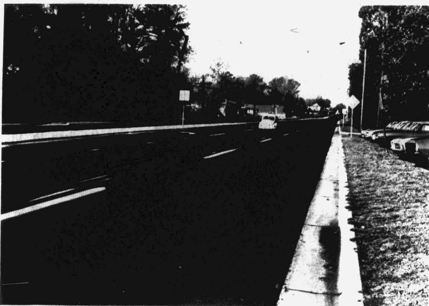
TENTH STREET PROJECT . . . The five-laning improvement on Tenth Street from Cotanche Street to the U.S. 264 bypass has been completed. Traffic
