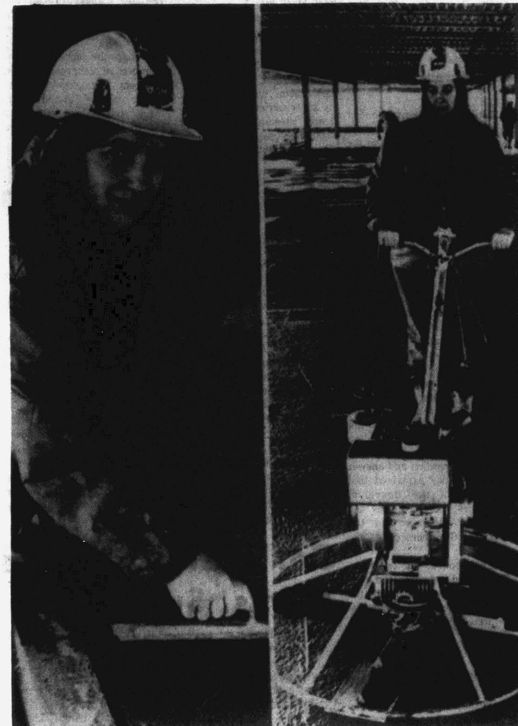
MOTHER'S JOB IS NOT IN THE HOME — Mrs. Naomi Huyard, only five feet, four inches tall, does a man's job as a cement finisher for a contracting firm at Lancaster, Pa. She traded
