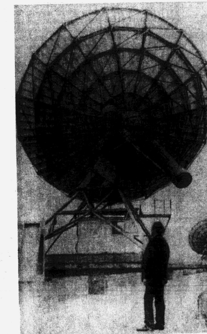
STRAIGHT TO THE STARS — Man looks at one of the eight new 42-foot diameter dish antennas comprising the five-kilometer radio telescope inaugurated at Lord's Bridge, Cambridge Tuesday. Most powerful of its kind, the new radio telescope was built for the British Science Research Council at a cost of $5.3 million. The steerable dish antennas are spaced on a line about 5 kilometers (3 miles) long. (AP Wirephoto)
