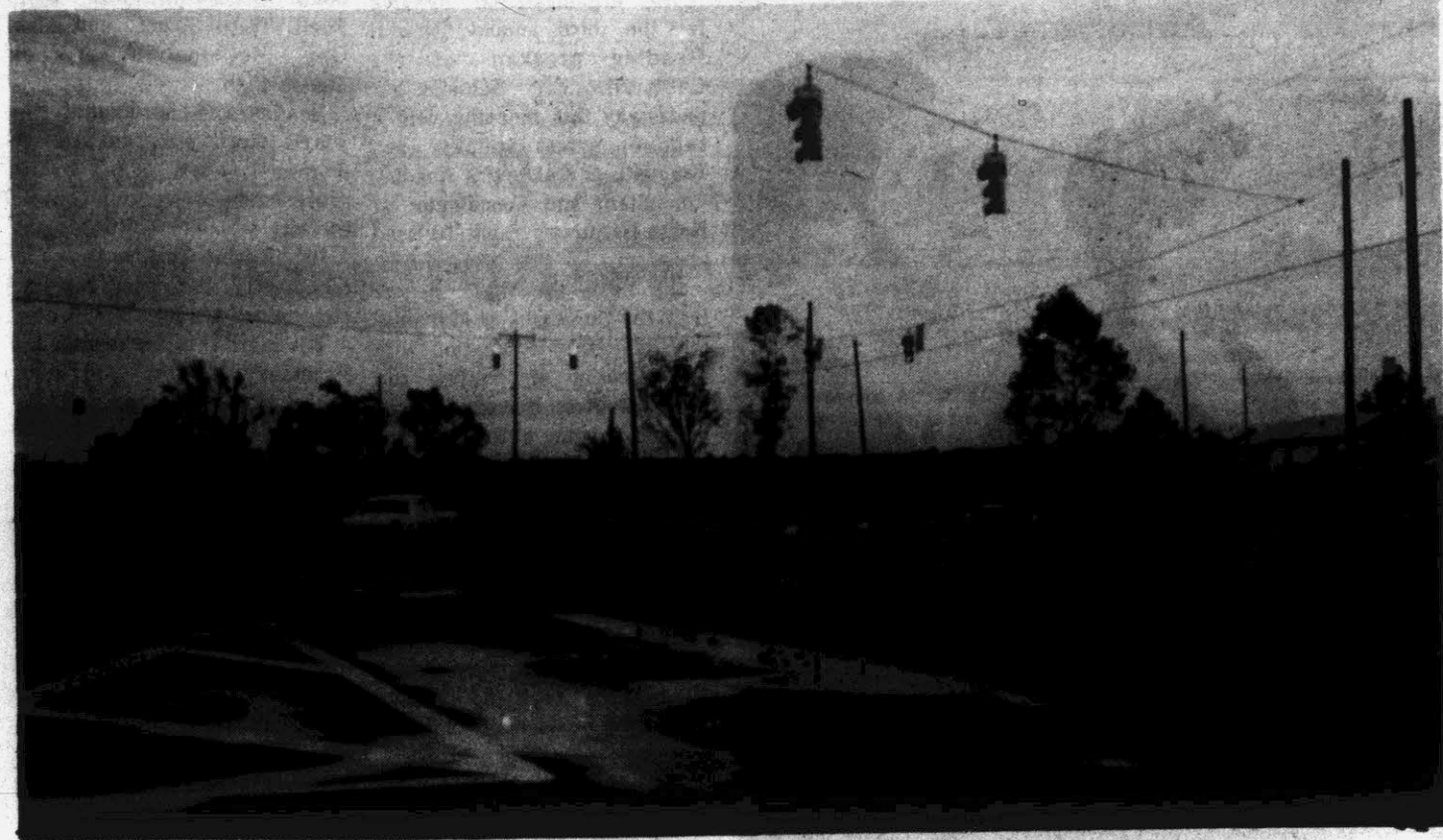
PROJECT COMPLETED — The Frog Level project, including 2.47 miles of work, has been completed. The project included widening of the two-lane highway to a five-lane roadway with curb and gutter. A traffic signal has been installed at the intersection of U. S. 264 business and U. S. 264 bypass. (Reflector Staff Photo)
