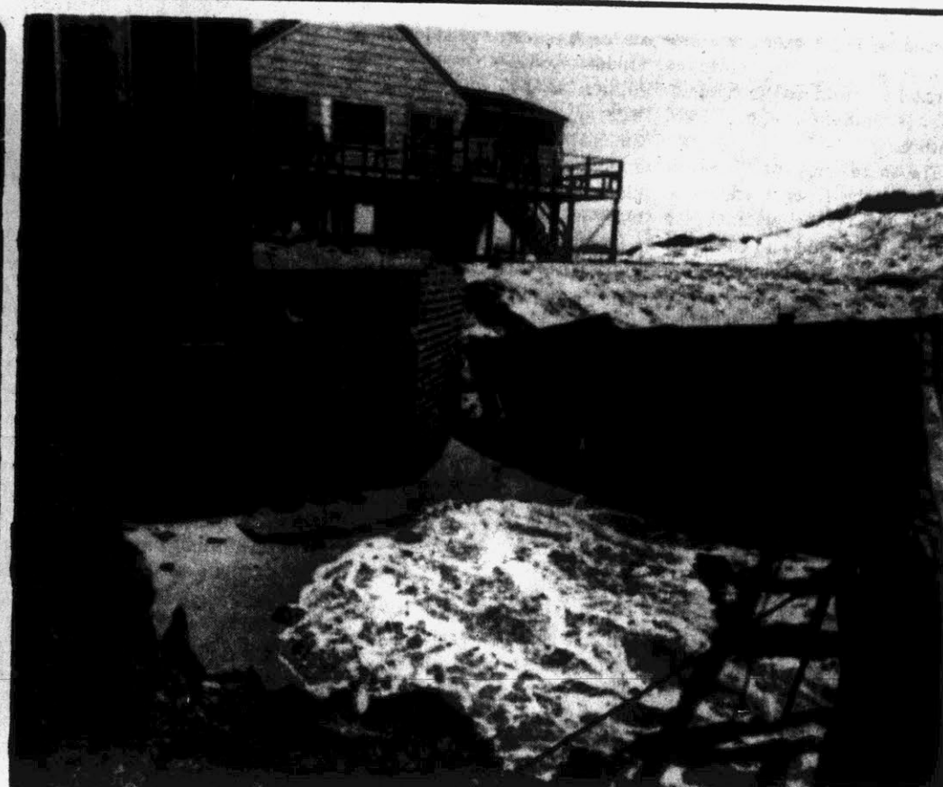
INCHING FORWARD — This sea wall was rebuilt after the ocean took part of the house, but a new wall is not faring much better. Here the tide is sucking the fill material from behind the wall. Note new house being built in background. (AP Wirephoto)
