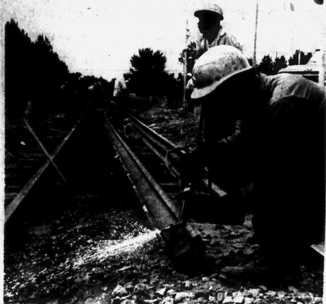
REWORKING CROSSING — Workmen lay new rails along the Elm St. Norfolk Southern railroad crossing yesterday, causing traffic to be rerouted into the opposite lane of the four-lane street for a short time. Workmen on the scene
