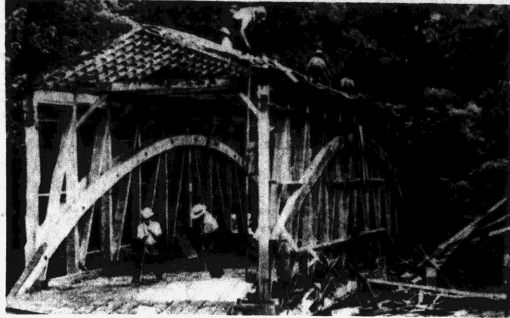
AMISHMEN DISMANTLE BRIDGE — A Lancaster County (Pa.) contractor and his hired help start dismantling the Pinetown Covered Bridge. The bridge, near Lancaster, was one of several covered bridges swept down-stream by
