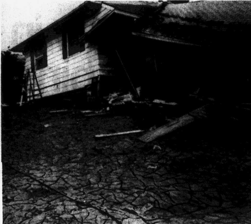
RESIDUE OF A FLOOD — A collapsed house and sidewalk are blanketed with a residue of mud left from the 20-foot flood waters that ravaged Wilkes-Barre, Pa. (AP Wirephoto)
