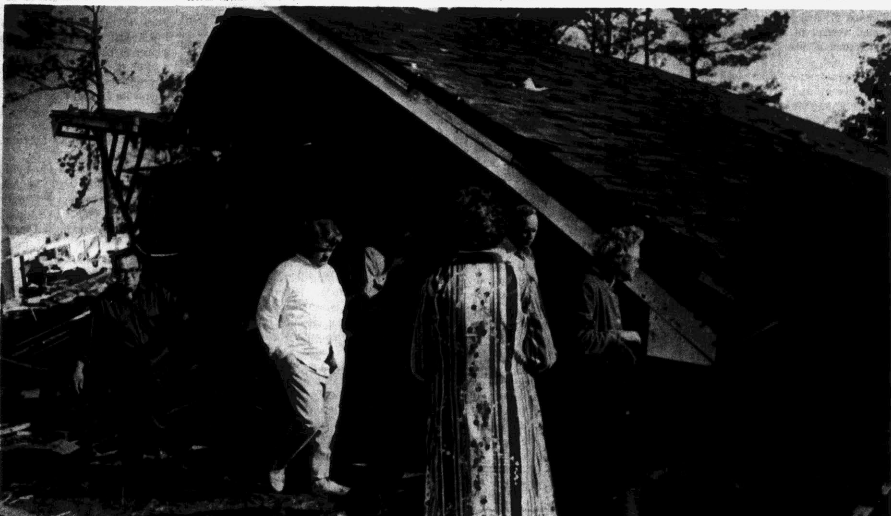
CHURCH MEMBERS SURVEY DAMAGE. ... Church members look over what is left of the recently built Red Oak Christian Church on the 264 by-pass. The church was totally destroyed during the storm. (Reflector Photo by Tommy Forrest)
