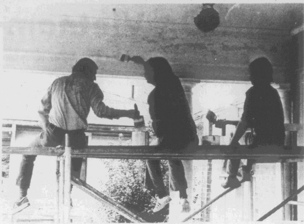
A TRIO .... of Phi Kappa Tau Fraternity members apply fresh white paint to the front porch of the Greenville Art Center. (Reflector Photo by Jerry Raynor)
