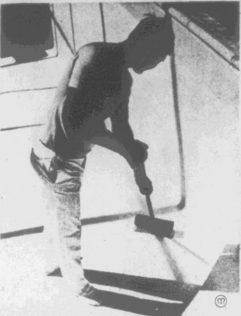
Remove protective winter covers from pool and equipment and sweep inside pool and surrounding areas. Inspect pool to determine if any cracking of walls or floors has occurred. And don't forget to examine all exposed valves, controls and pipes.
