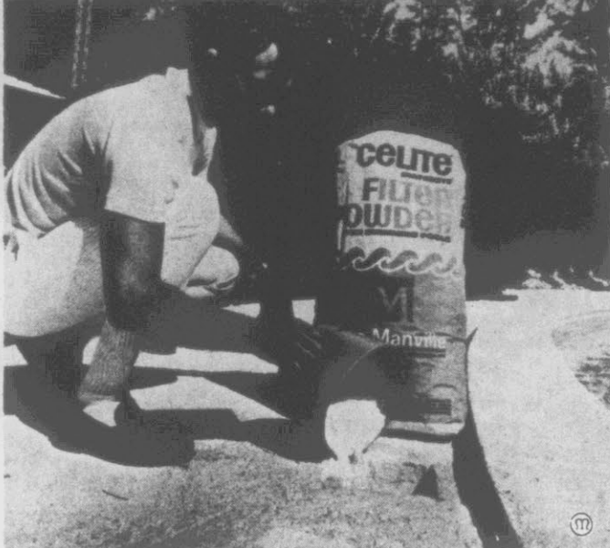
Proper precoating of filter elements with filter aid assures crystal clear water. This is done by circulating a mixture of diatomite and water into the filter to provide a coating about 1/16" thick on the elements. As filtration progresses, the improved clarity and sparkle of water will be amazing. Chlorination and the addition of other chemicals or algicides is the next step. Now for the first dip... weather permitting.
