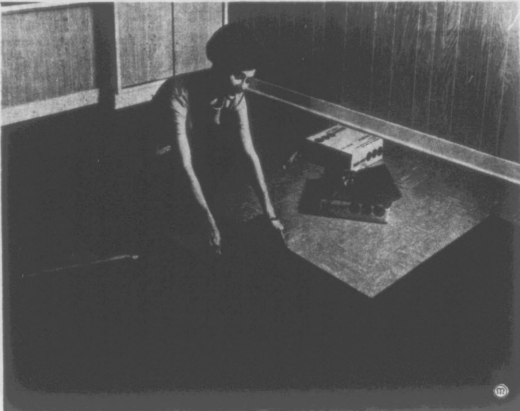
Covering an old kitchen floor is fast and easy, thanks to new self-adhering vinyl-asbestos tiles from Armstrong. Each tile comes with the adhesive already applied to the back. To install, simply peel off the protective paper backing, set the tile in place, and press! It's easy enough for the home maker to do herself.
