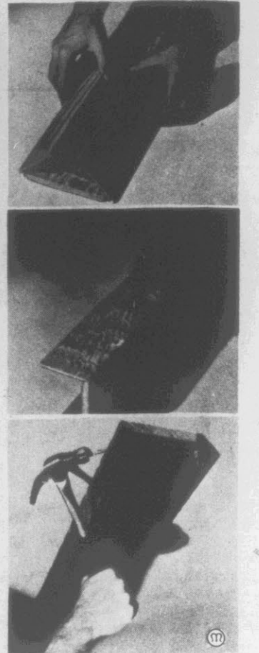
Growth of the trend toward more casual living and the craze for Country Western have inspired an innovative plywood beam system making it easy to achieve decor such as that pictured above. Weldwood hand hewn beams are manufactured in three sections attached with cloth strips (upper right). Assembled and nailed at joints to form a U channel (center right) the "beams" are ready for nailing to a previously installed nailer strip (below). They may be natural, painted or stained. Photos from U.S. Plywood.
