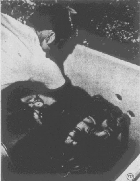
If all seems proper, turn on water to fill the pool. Again examine all valves, controls and pipes for leakage. While pool is filling, check filtration equipment for operational readiness. Follow manufacturer's cleaning directions.
