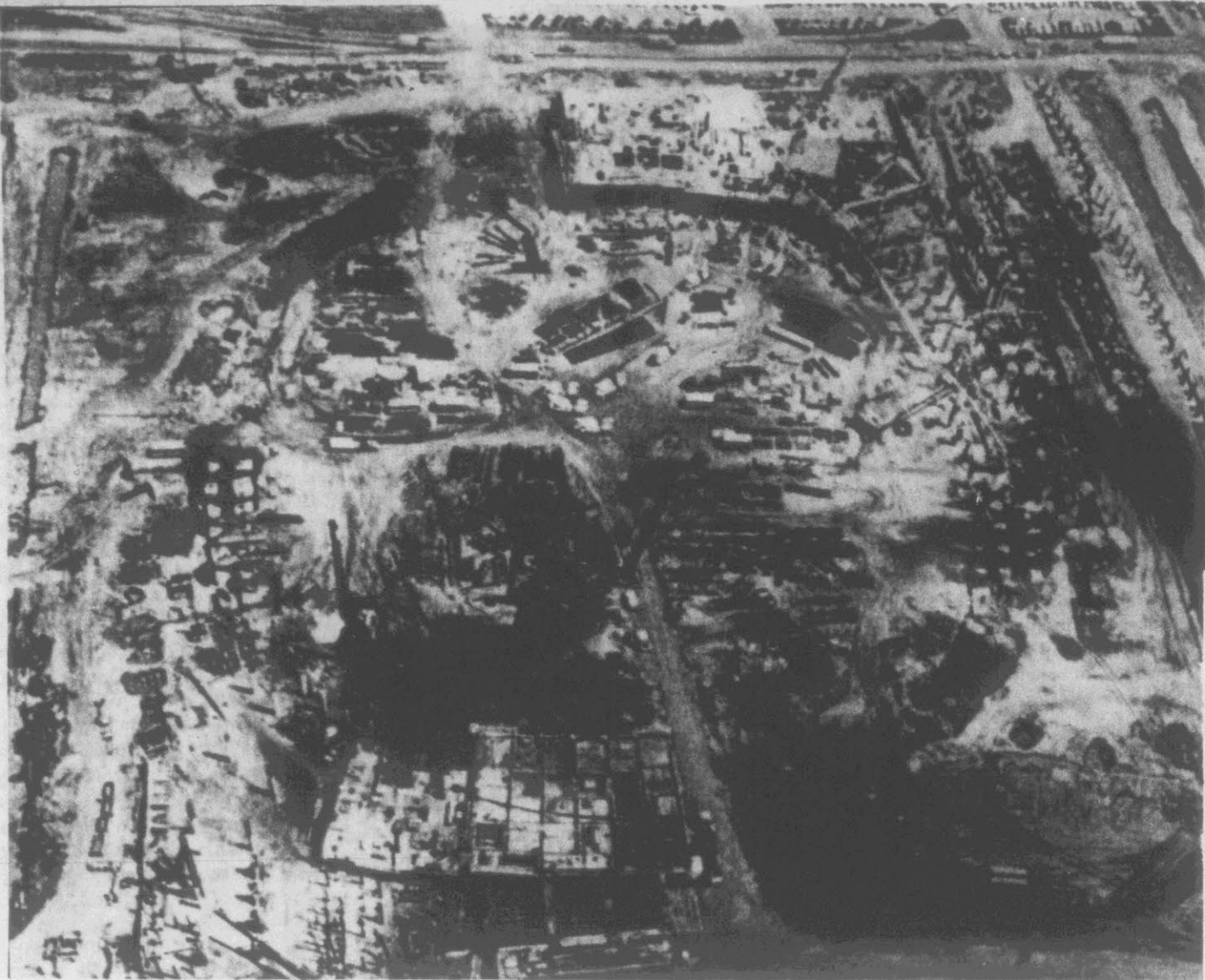
Future Major Sports Arena DOME TAKING SHAPE — The $124.5 million Super Dome in New Orleans is beginning to take shape as revealed in this aerial view. The foundation of the dome, which has been criticized as inadequate, was said to be the only safe and practical way to construct the building. (AP Wirephoto)
