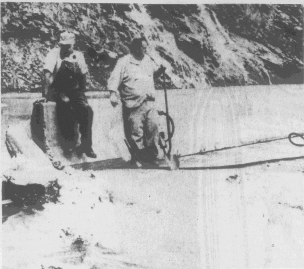
THIS IS A HIGHWAY? —Workmen 'watch backed-up water pour through a hole in a dividing barrier on Interstate 40 near the North Carolina-Tennessee line. Water and dirt blocked portions of the highway in Tennessee and North Carolina. The area pictured is on the North Carolina side, about a half-mile from the border. (AP Wirephoto)
