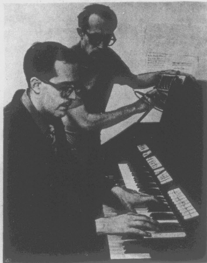
COMPUTER ORGANIST — Dr. Alan Ashton, University of Utah computer scientist, and Robert Bennion, computer student, operate an organ connected to a computer. A tune is played on the organ and recorded in the computer, which plays it back, changing volume, speed, key and correcting any errors in the recording.
