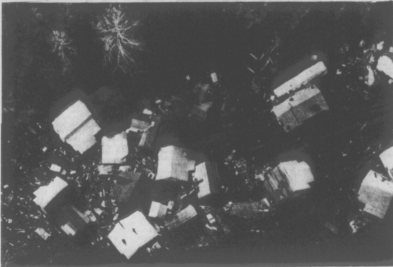
FLOOD DEVASTATION — Houses in Craneco, West Virginia, are flung together the day after a flash flood killed at least 60 people. (AP Wirephoto)
