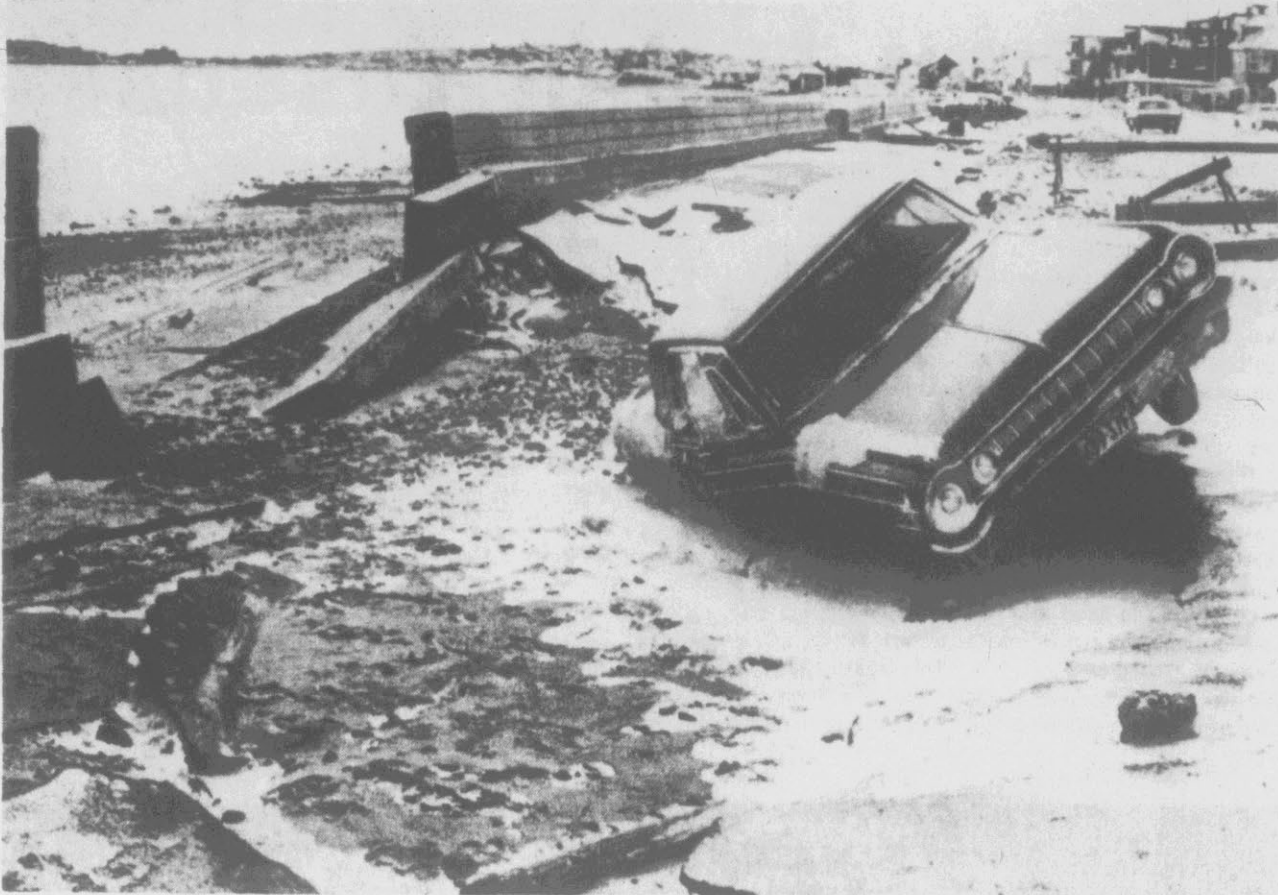
SEAWALL SMASHED — Giant waves driven by the worst storm of the winter to strike New England swept through the seawall at Revere Beach undermining roadway under this car. High tides,
