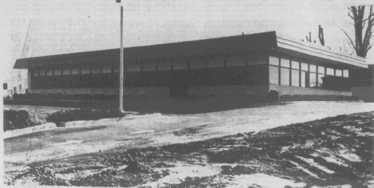
NEW BNC OFFICE...The finishing touches are being added to the Bank of North Carolina's new office on E. Tenth Street in preparation for Thursday's opening and dedication activities. The structure, con-
