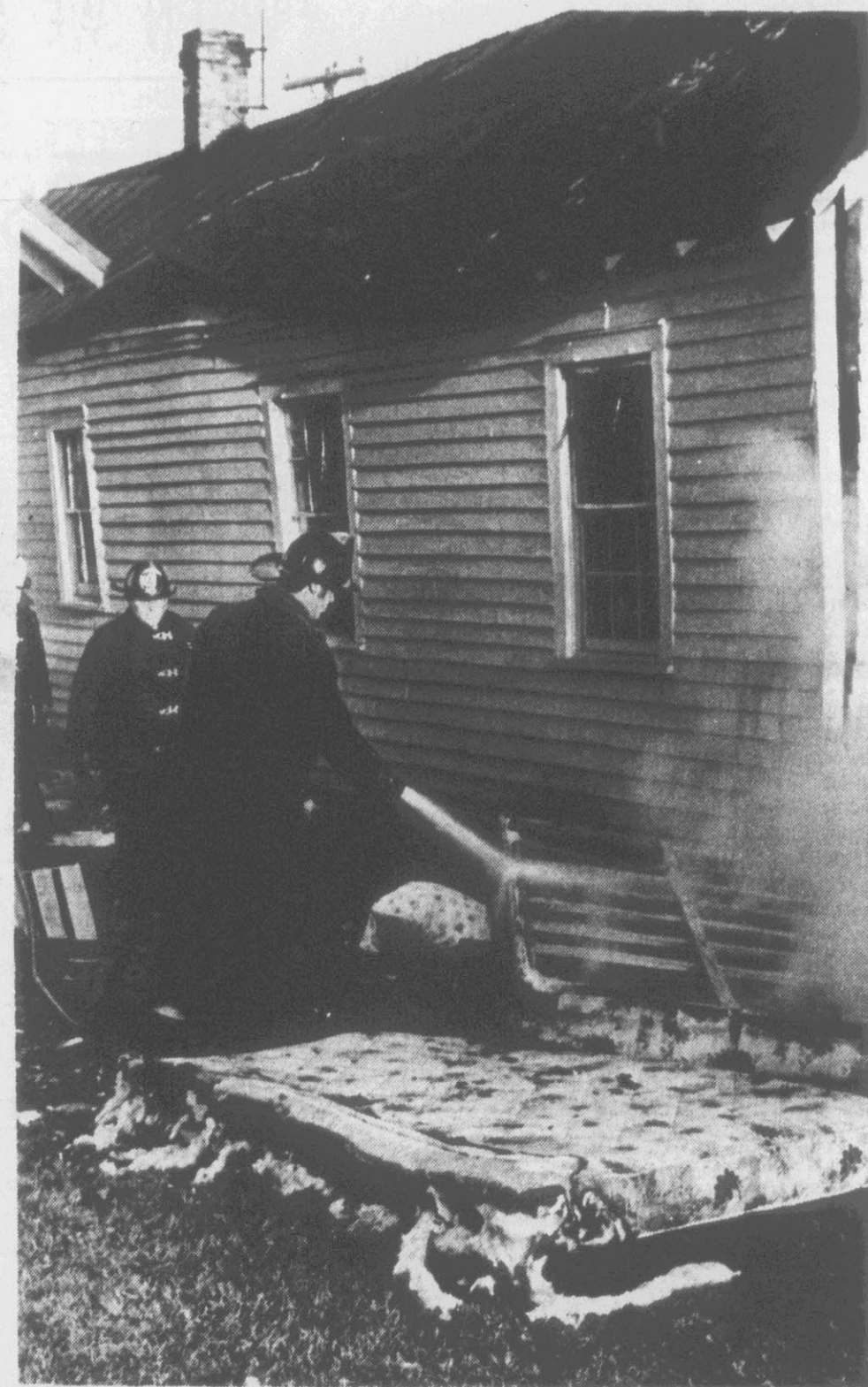
HOME RIPPED BY EXPLOSION ... Firemen cool a mattress after a gas explosion in a home on 14th Street. The home was blown apart from the intense
