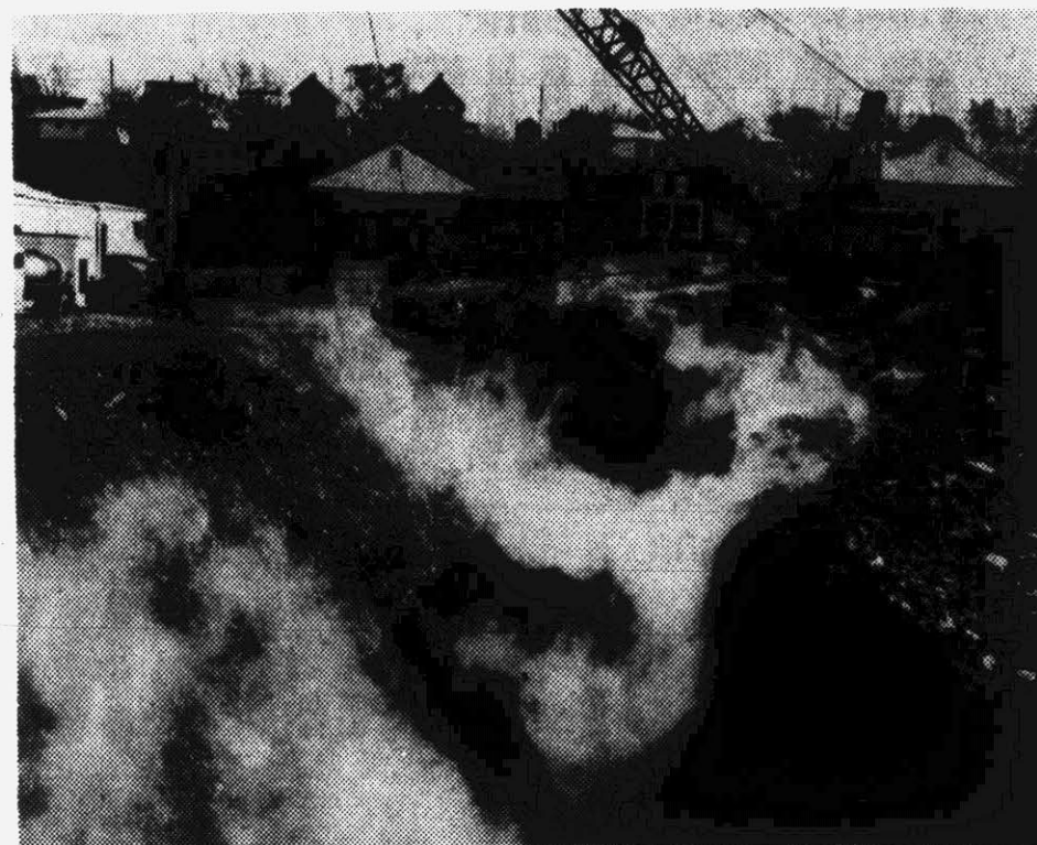
A trench is dug to try to cut off underground fire; but it smokes on.
