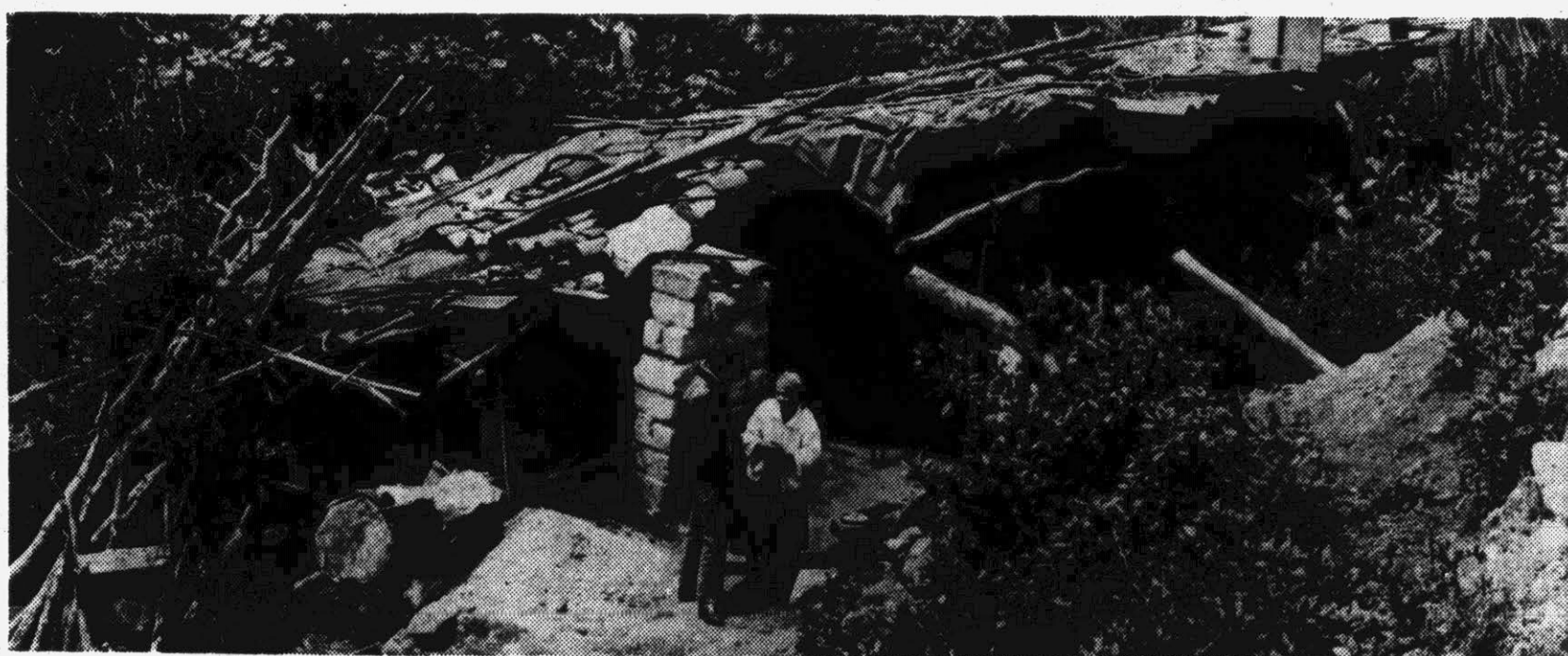
...most of the community's buildings have only been shacks such as these up to now.
