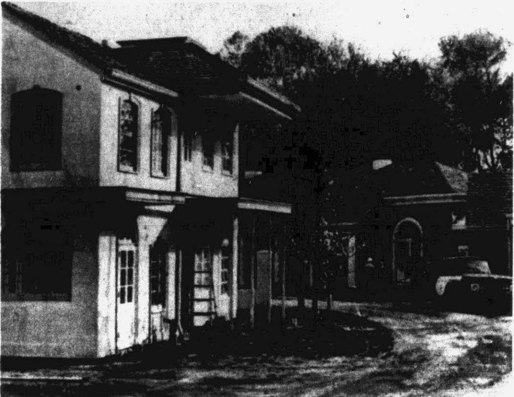
AMERICAN JAZZ AND BLUES AREA — Workmen are putting finishing touches on the many buildings of the American Jazz and Blues area, which will highlight the music that came out of New Orleans. (AP Wirephoto)
