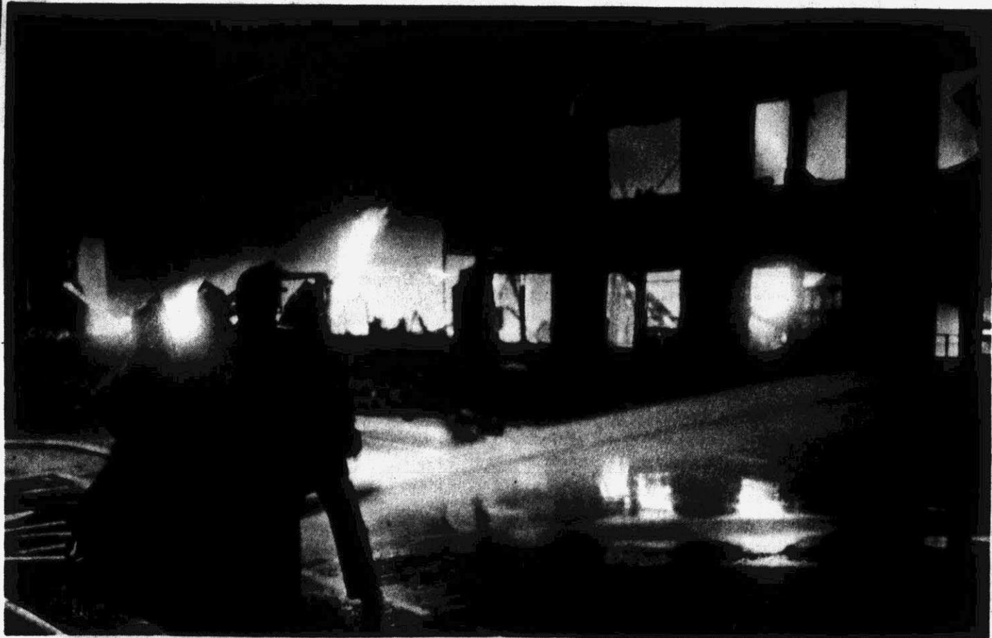
WAREHOUSE DESTROYED... Farmville firemen leveled the building which housed the smallest tobacco auction operation in Farmville. play stream of water on fire at Lee's Warehouse on South Main Street last night. The 10:30 p.m. blaze
