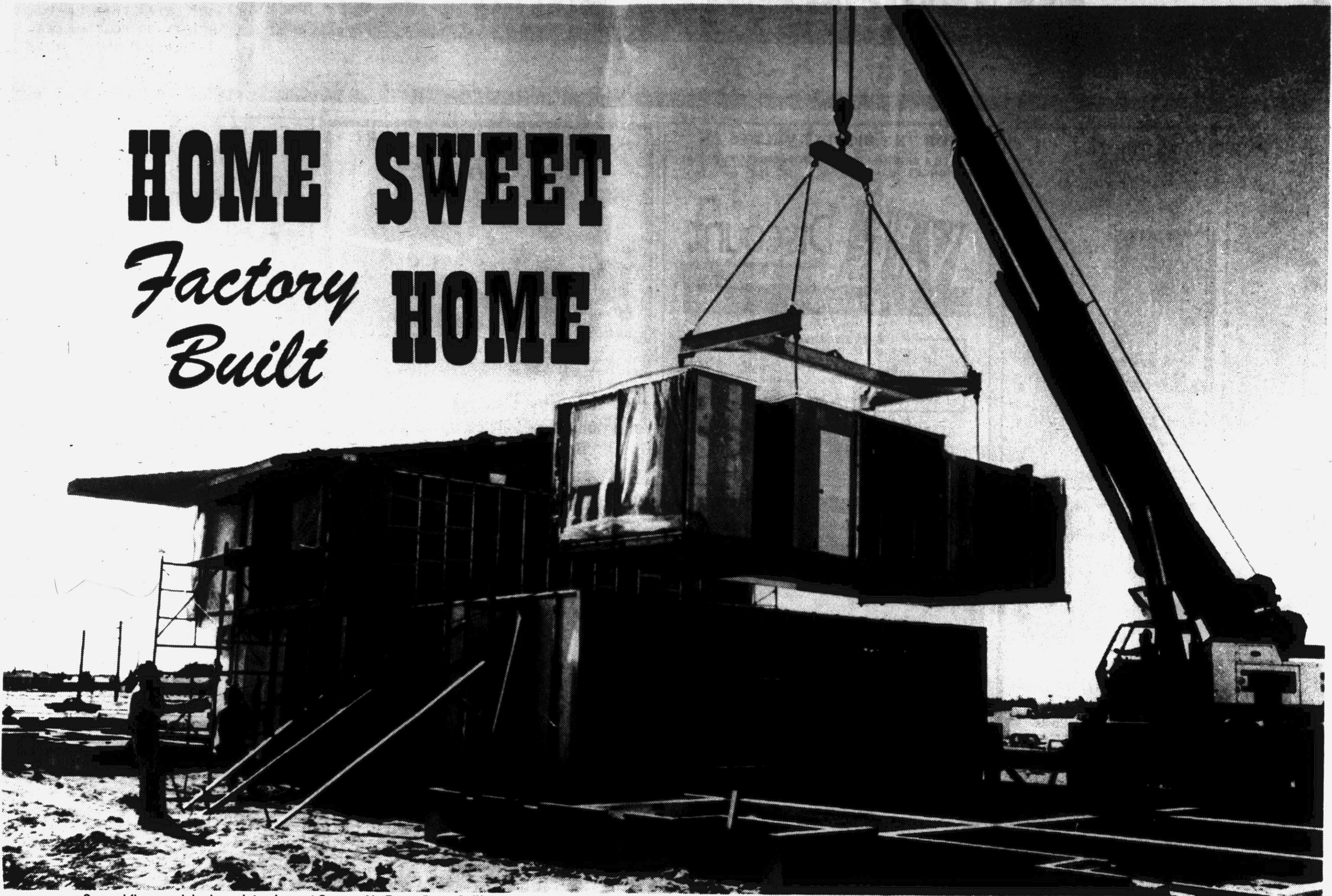
Second floor module drops into place at George Air Force Base, Calif.
