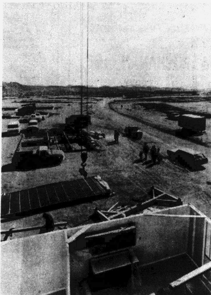
Modules are quickly put together on the site . . .
