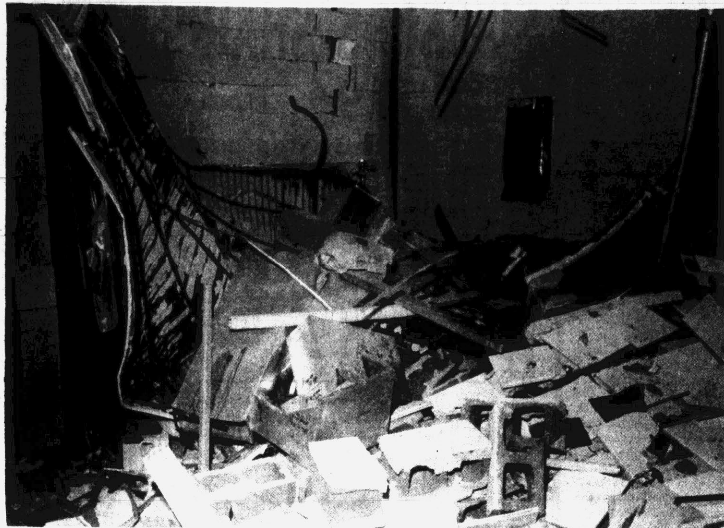
AYDEN-GRIFTON SCHOOL DAMAGE . . . debris occupies what used to be a rest room at the rear of the new school's auditorium. Workmen completed work on the auditorium about 20 days ago. None of the 800 students or 47 staff members were injured. (Reflector Staff Photo)
