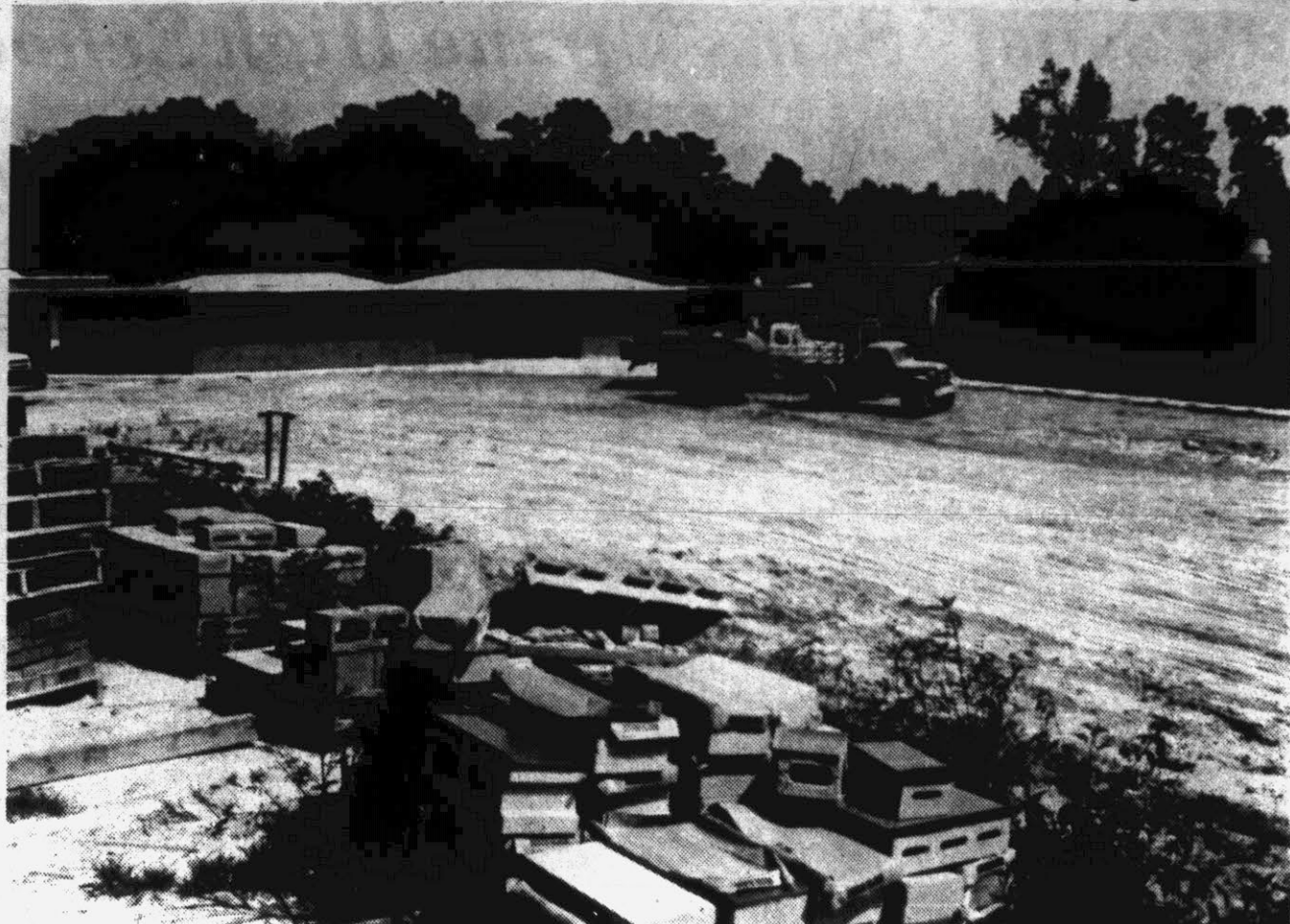
TAKING SHAPE . . . The low single story units of the new Wahl-Coates Elementary School comes into the construction homestretch as school time draws near.
