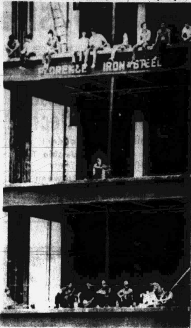
ALL ALONE —Construction workers at the new Merchandise Mart in Charlotte take time out for some lunch, fellowship and, possibly, girlwatching. All except the fellow on the middle floor. He didn't get in on the fellowship. (AP Wirephoto)
