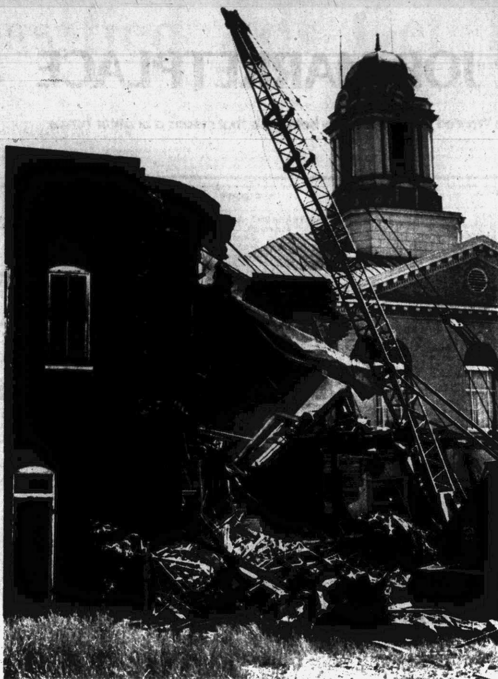
DEMOLITION . . . The rear portion of the Edwards Building is the target of the heavy wrecking ball as workmen from Chapel Hill pressed the demolition of the old brick structure. By this morning, most of the building had been torn down. (Reflector Photo).
