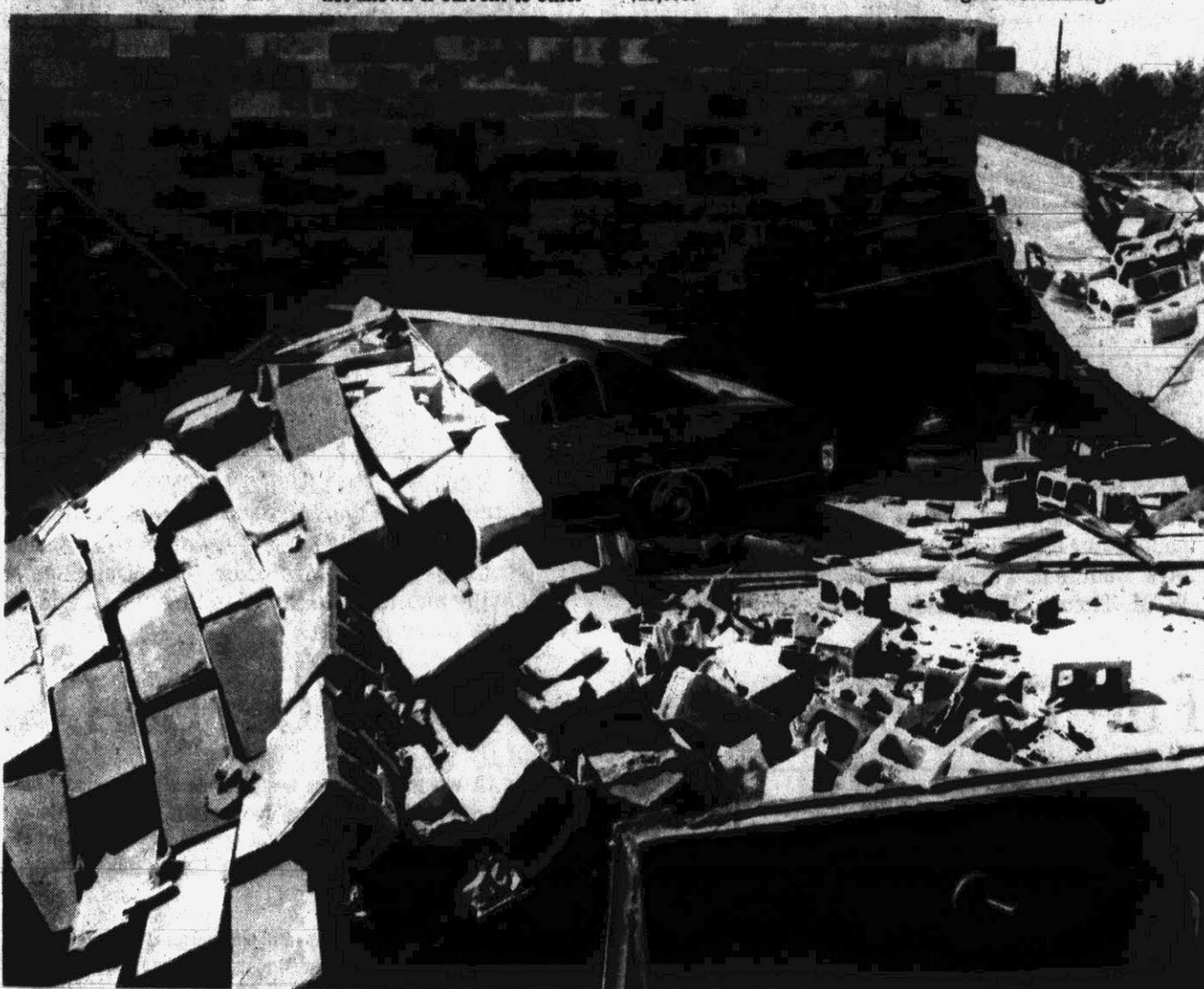
BODY SHOP DESTROYED NEAR GRIMESLAND ... Dixon's Body Shop near Grimesland suffered heavy damage as a result of the high winds yesterday
