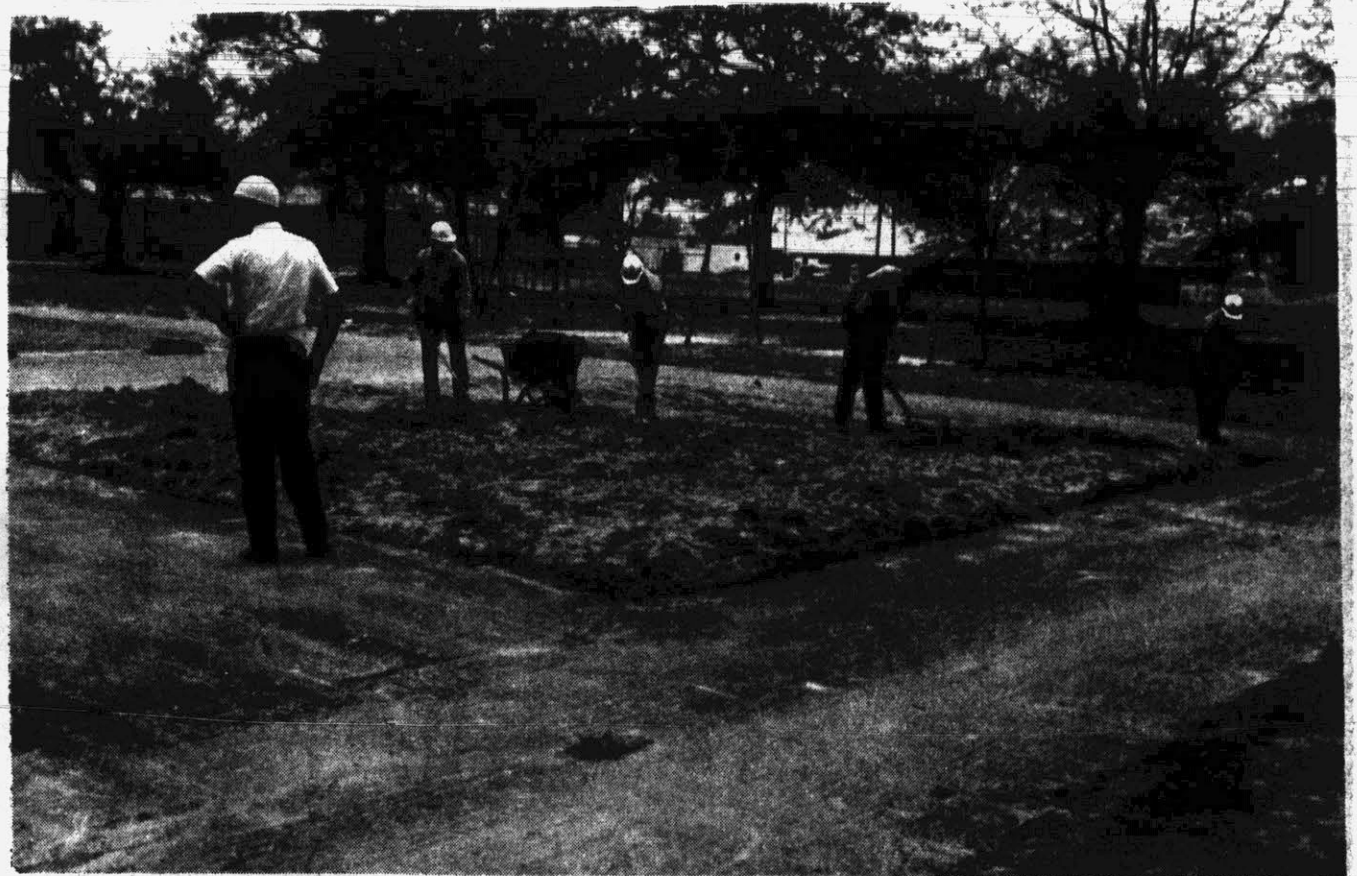
CITY WORKMEN . . . prepare the site for Safety Town.
