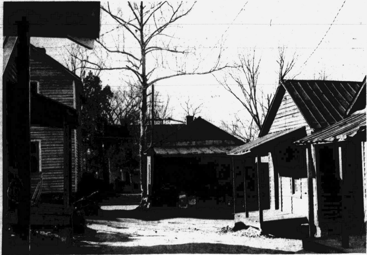
Shore Drive Area As It Was Before The Urban Renewal Project!
