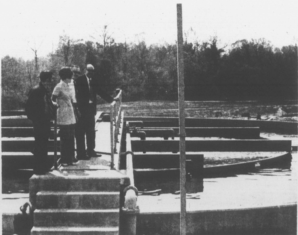
THE GREENVILLE WATER POLLUTION CONTROL PLANT . . . is visited by Mrs. William Fore. Shown with her are Rex Voorhees, superintendent of water and sewer depart-
