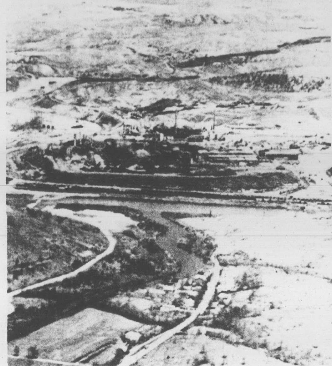
THE TENNESSEE SAHARA — A large industrial complex, the Cooperhill Operation of Cities Service
