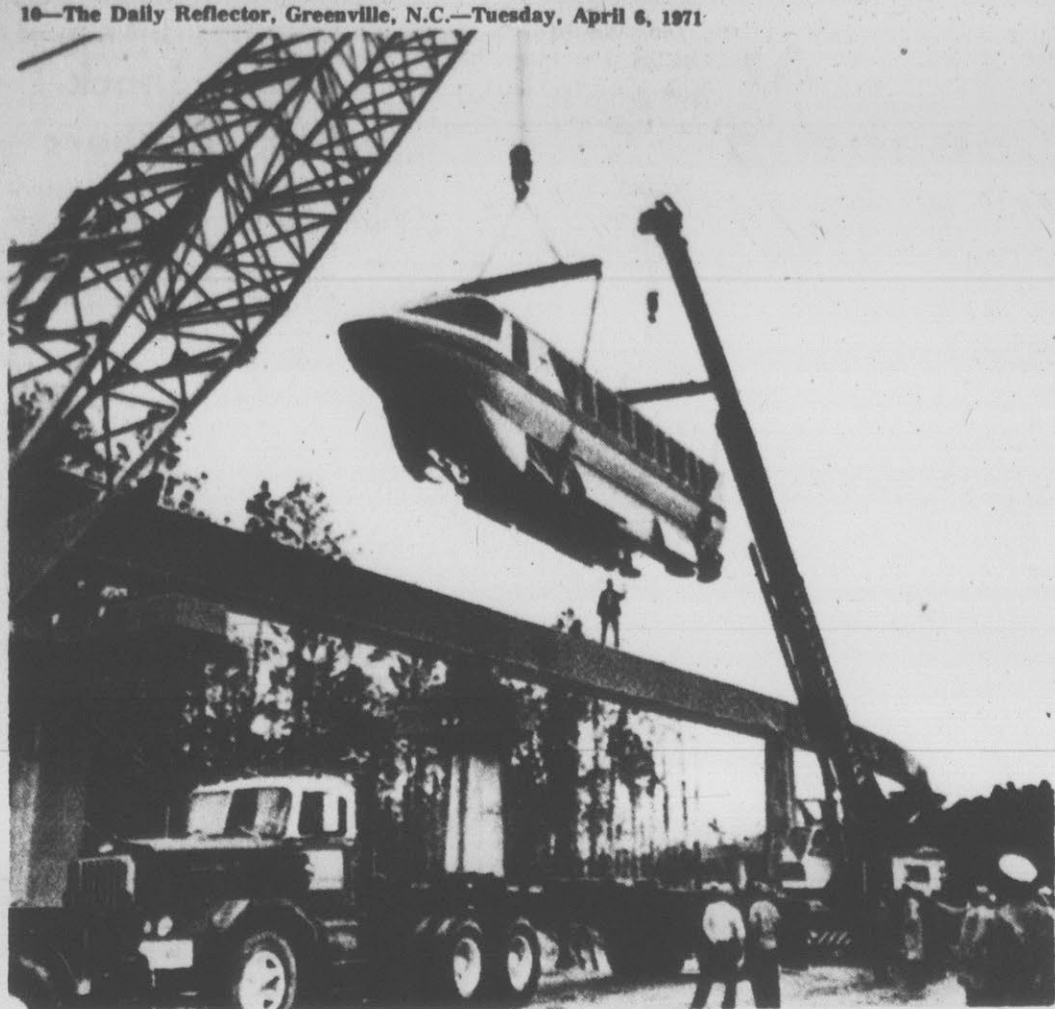
MONORAIL READIED —Work crews hoist a monorail car atop 20-foot high beamway at Disneyworld vacation kingdom. System spans three miles and will be main mode of transportation, stopping at each of two hotels on the
