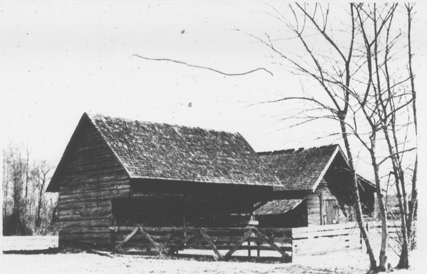
AN OLD MULE STABLE . . . with an overhang front was a common type of construction in the 19th century. This one, with its original split shingles, is on the Rogers Farm on the Wild Cat Road near Williamston.
