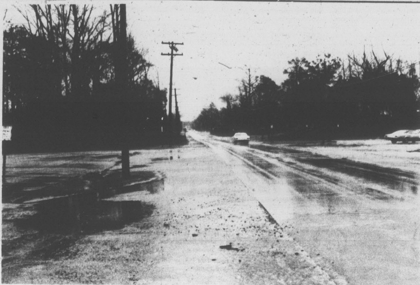
TENTH STREET IMPROVEMENTS... bids have been called for on improvements to Tenth Street from
