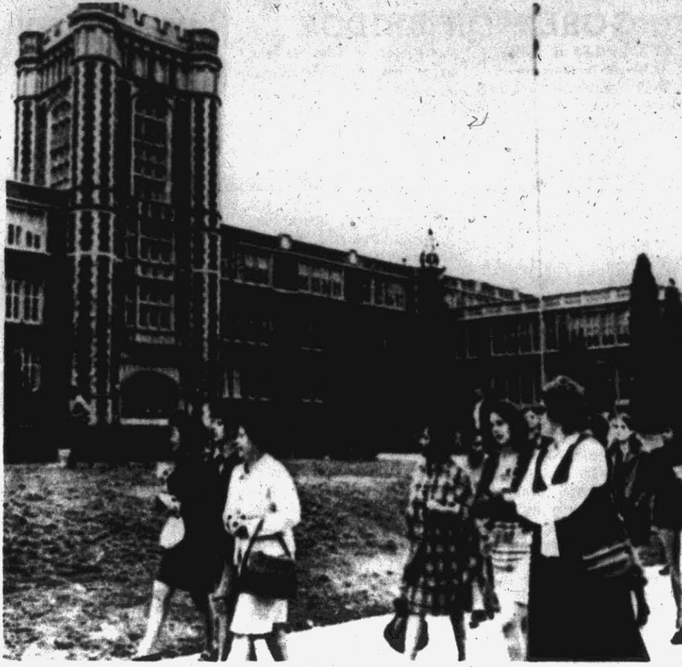
SCHOOL CONDEMNED — The Los Angeles High School, the city's oldest and best known, was condemned Tuesday because of earthquake damage. It is familiar to television viewers as the background setting for the network series
