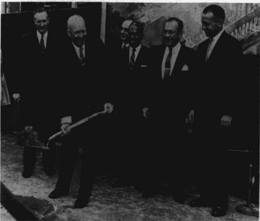
President Eisenhower breaks ground in May, 1959, and Lincoln Center for the Performing Arts begins to become a reality.
