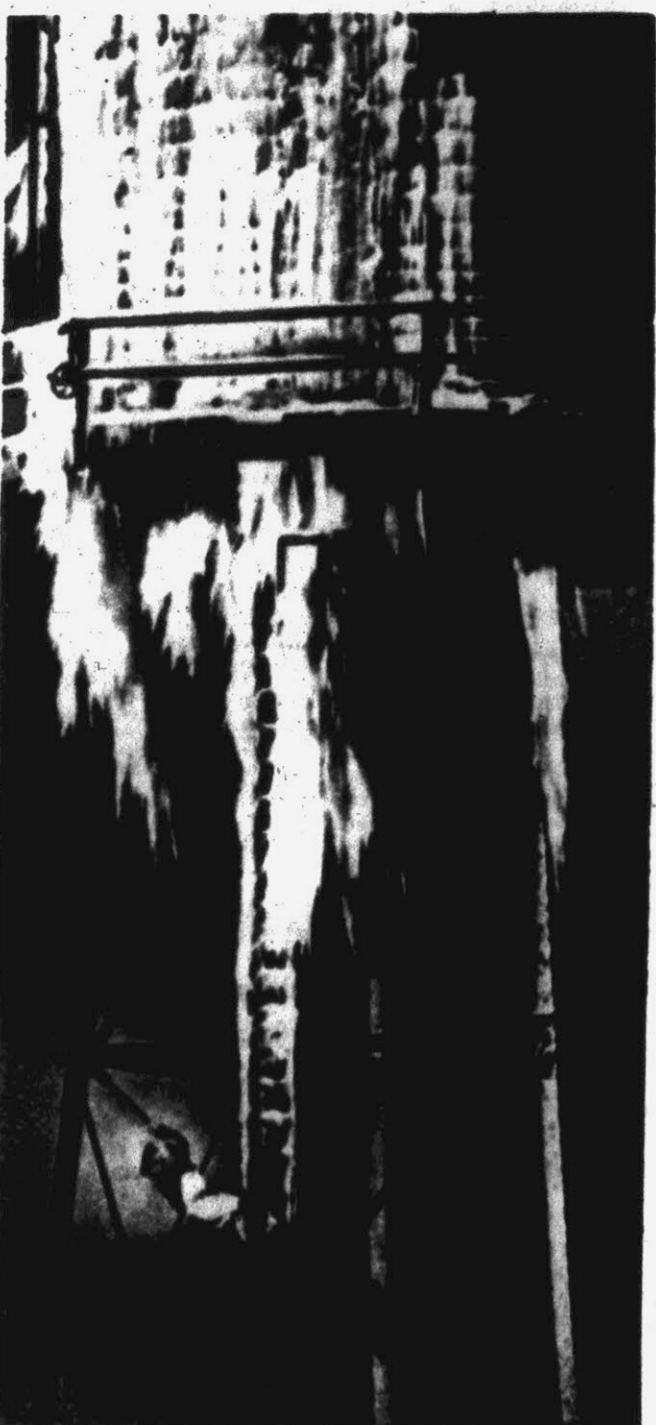
COLD HANG-UP — Elwin Tiffany, a welding company employe hangs precariously 60 feet in the air in an attempt to dislodge sheets of ice hanging from a burst water tower in Mystic, Conn. The burst is a result of continuing cold weather. (AP Wirephoto)
